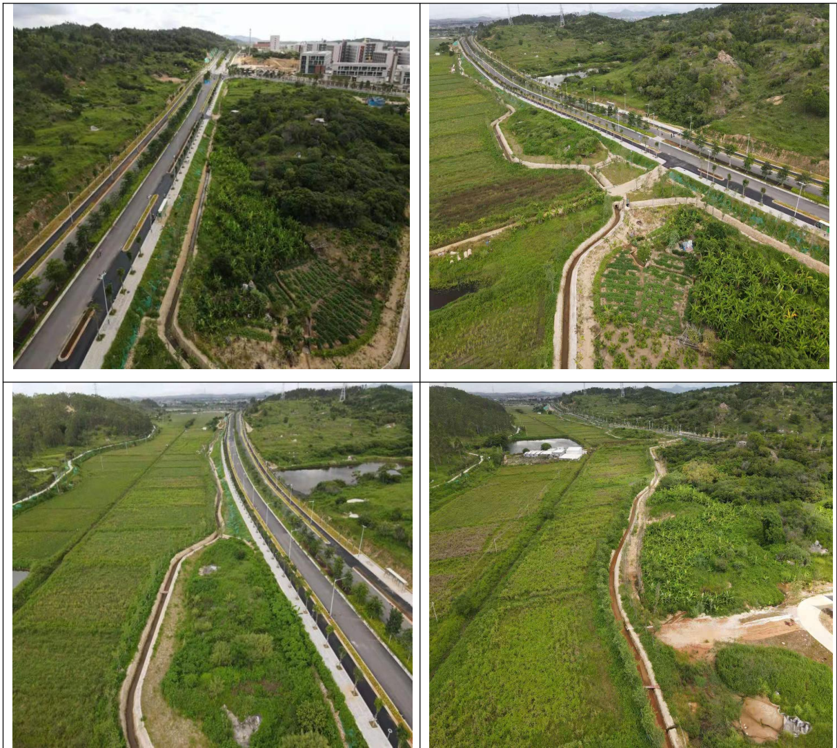
渠道改道区现状照片
